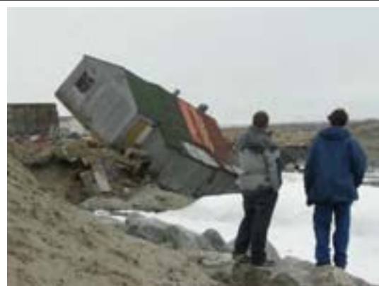
Figure 2-11. Damaged infrastructure in an Alaskan coastal community. This represents the juxtaposition of problems caused by increasing temperatures: permafrost melt destabilizing the ground combined with increased water temperature that reduces protective ice cover and allows waves to melt the base of permafrost bluffs and increase coastal erosion. Photo by Ned Rozell, Geophysical Institute/University of Alaska Fairbanks.
